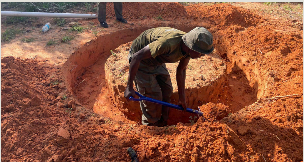
Digging the foundations for a water tank in our Reserve
